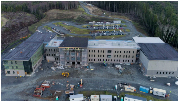
Above: Construction of new Seaside High School
