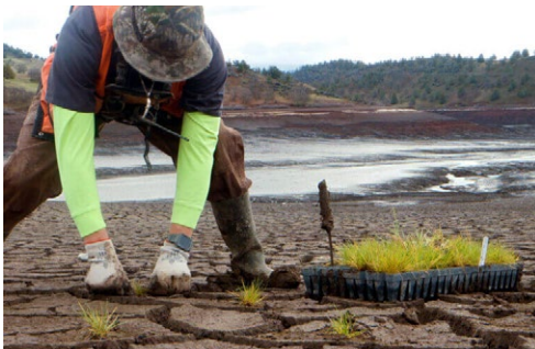
Replanting in the reservoir footprint post-dam removal.
