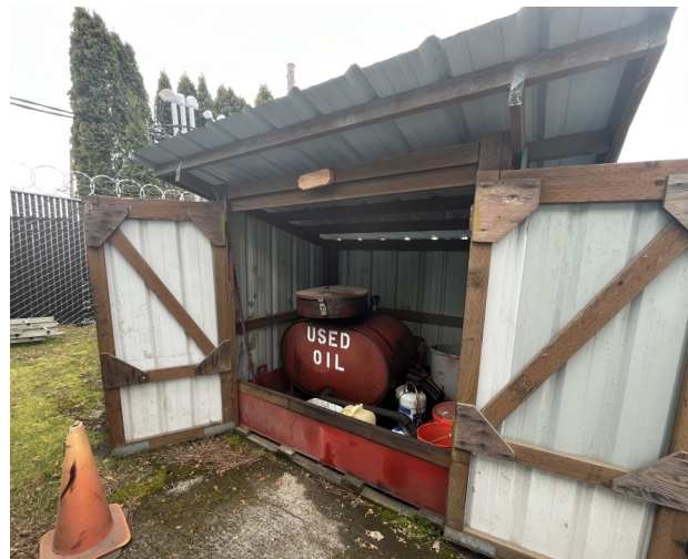
Used oil collection shed
