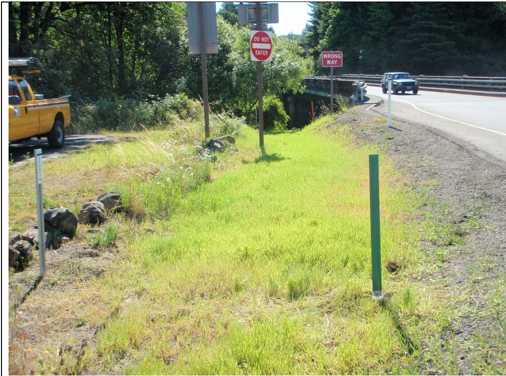
Figure 17-5 Stormwater Facility Field Markers (Swale along Hwy 22)
