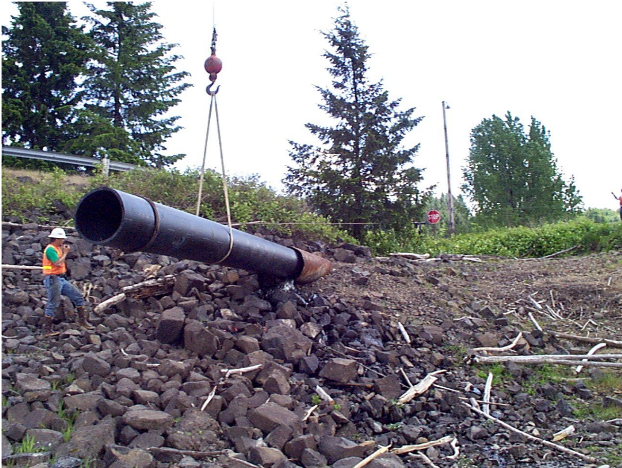
Figure 16-1 Sliplining with Fusion-Welded Continuous Pipe
