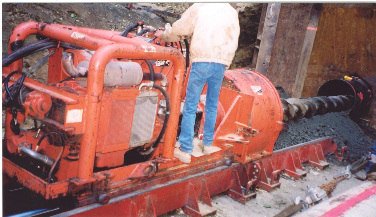
Figure 16-6 Auger Boring
