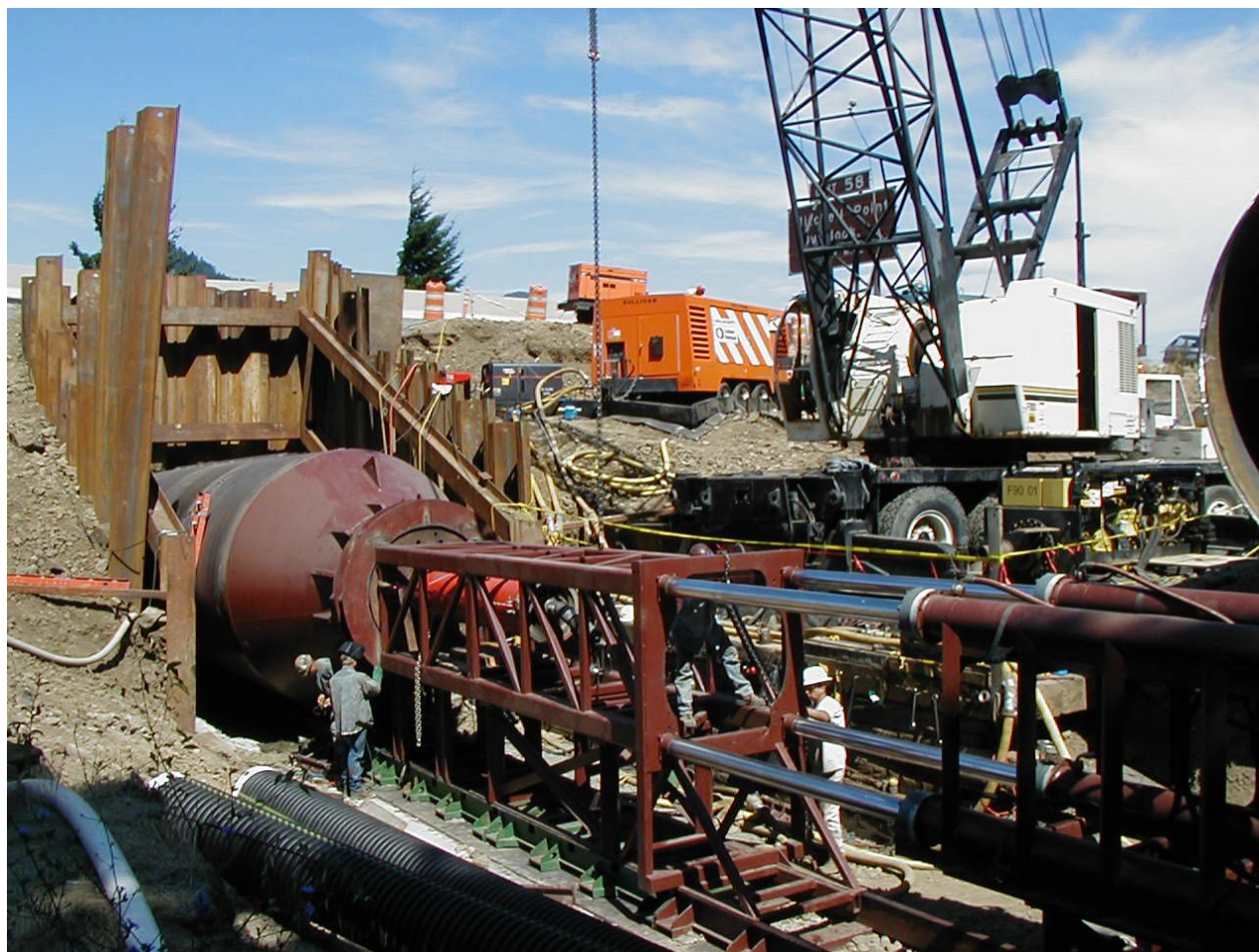
Figure 16-7 Pipe Ramming
