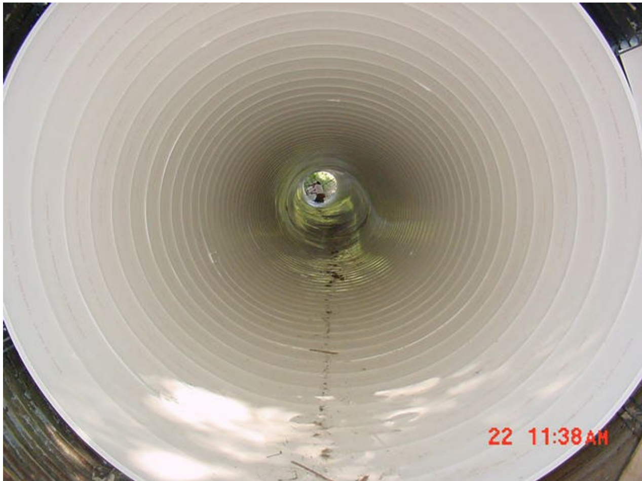
Figure 16-4 Spiral-wound pipe
