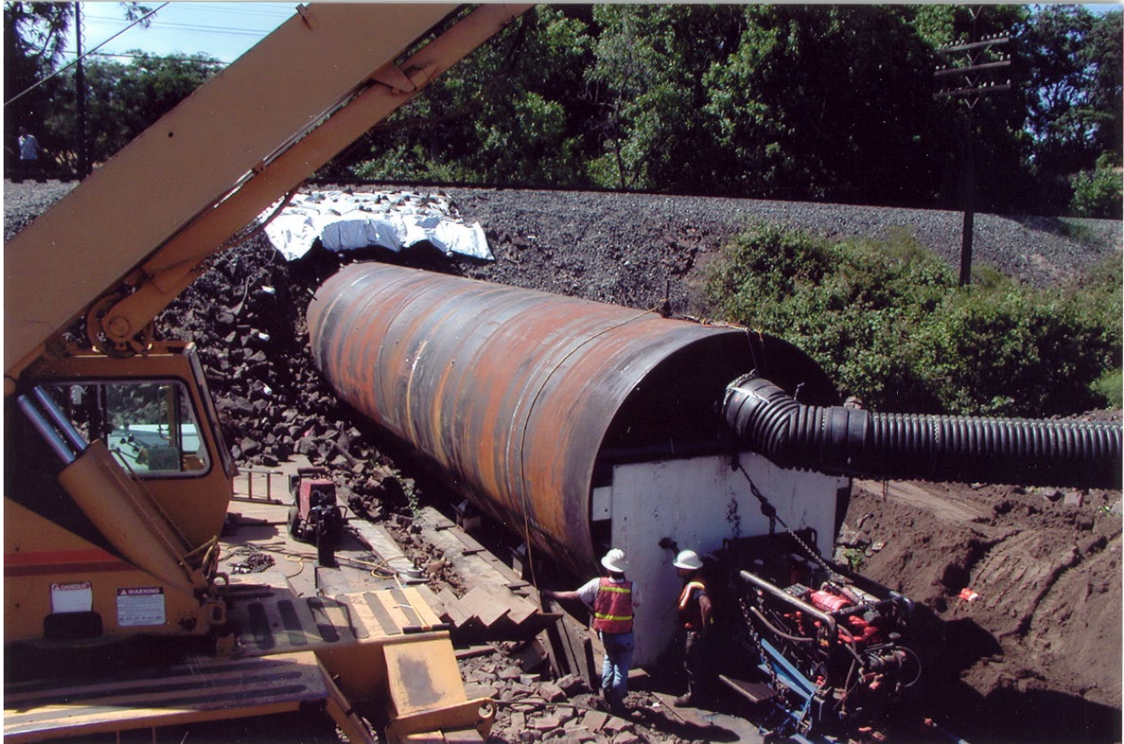
Figure 16-5 Pipe Jacking
