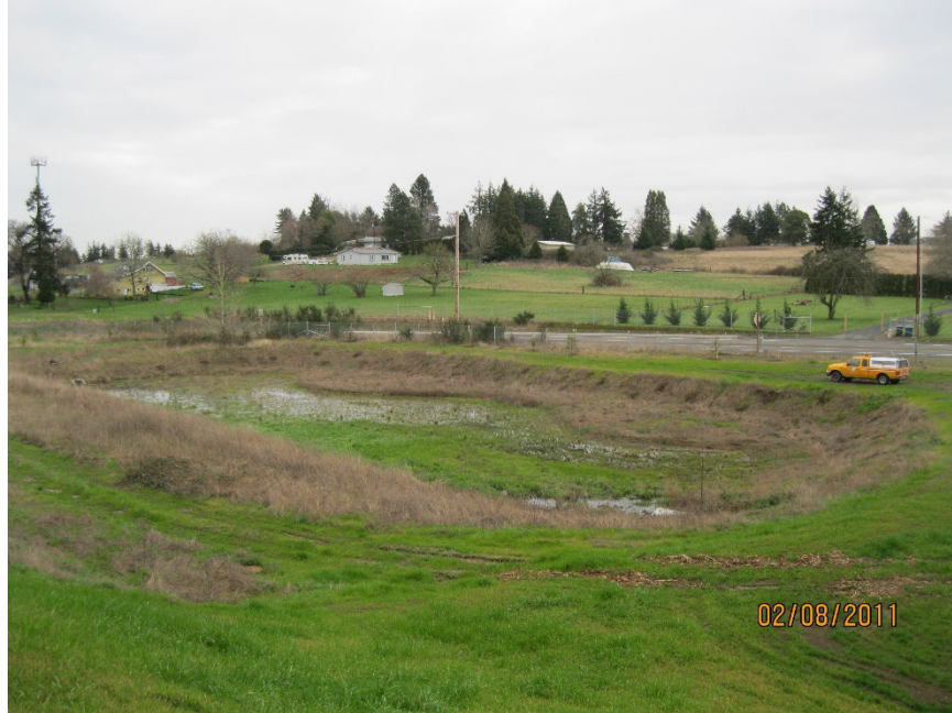
Figure 14-2 Combined Biofiltration Swale/Detention Pond
