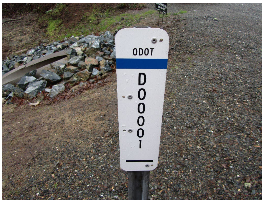
Figure 14-8 Stormwater Facility Field Marker (Type S2)
