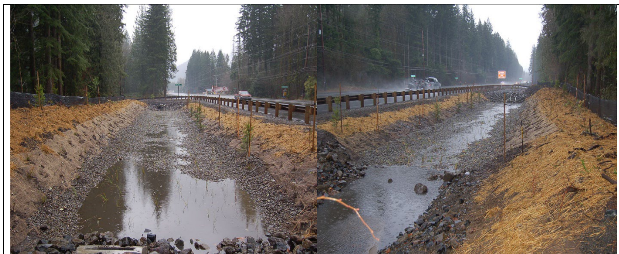
Figure 1 Extended detention dry pond
