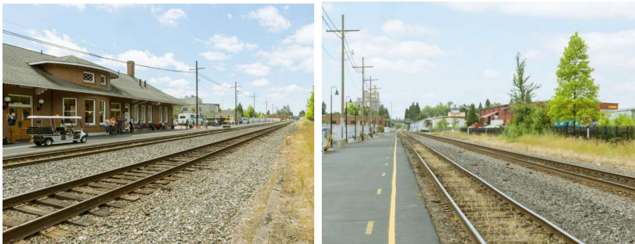
Figure 2. Photos of Existing Eugene Station and Tracks
