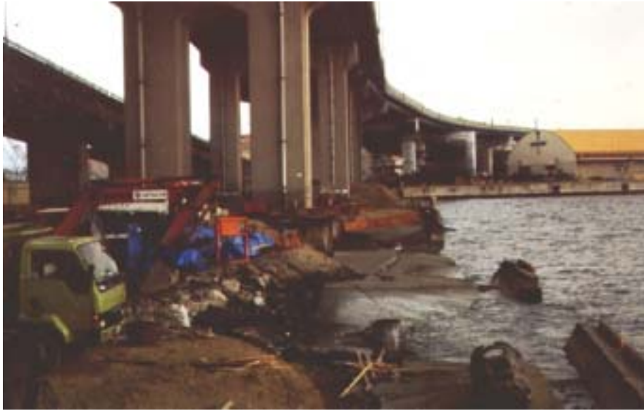
Figure 2.28: Dai-ni Maya Ohashi Bridge
