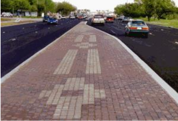
FIGURE 8-21 UNIT PAVERS IN MEDIAN
