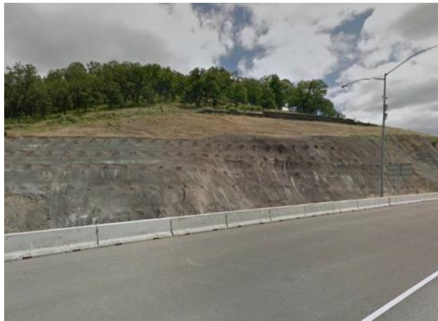
FIGURE 8-6 SHOTCRETE AND SOIL NAIL WALL ON I-5
