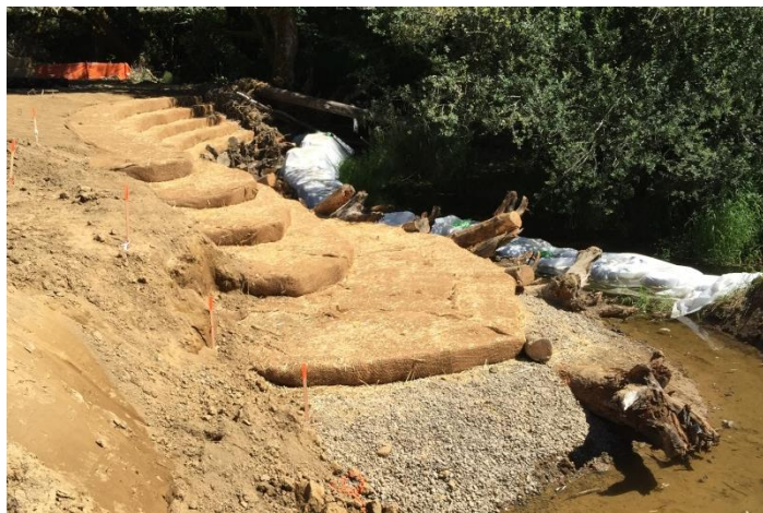
Figure 2-5 Matting Product Provides Protection of Waterway from Erosion
