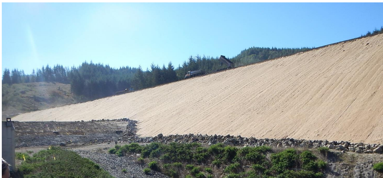
Figure 3-10 fully biodegradable slope protection matting
