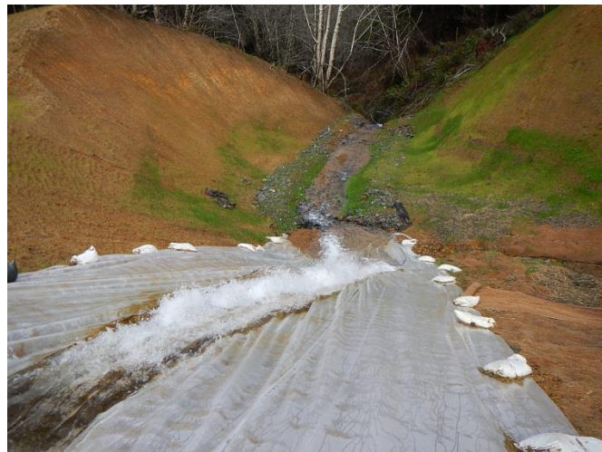
Figure 3-15 Plastic sheeting used as Temporary Slope Drains
