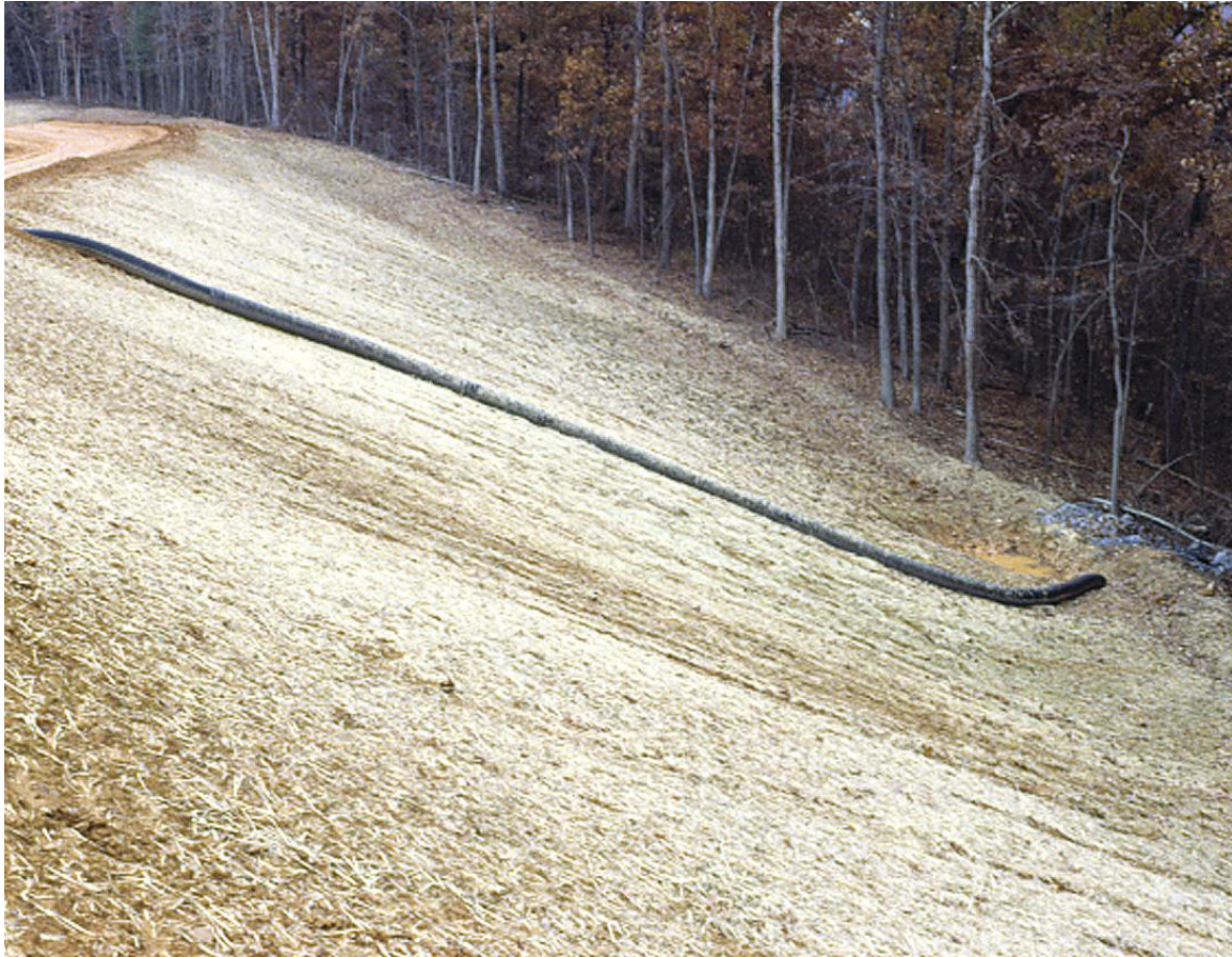
Figure 3-14 Temporary Slope Drains
