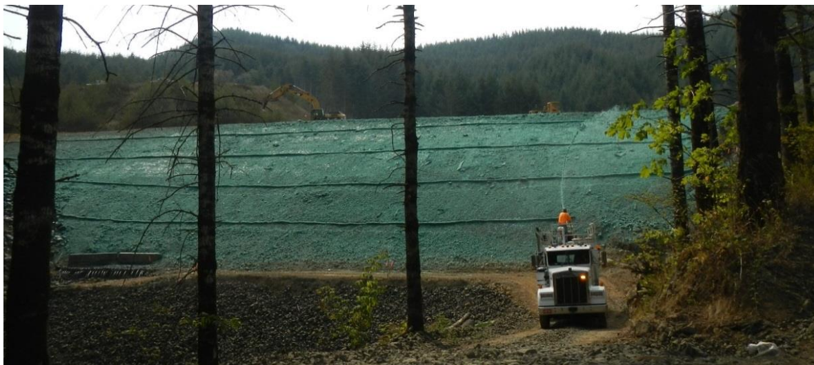
Figure 3-4 Seeding & mulch applied with Hydroseeder
