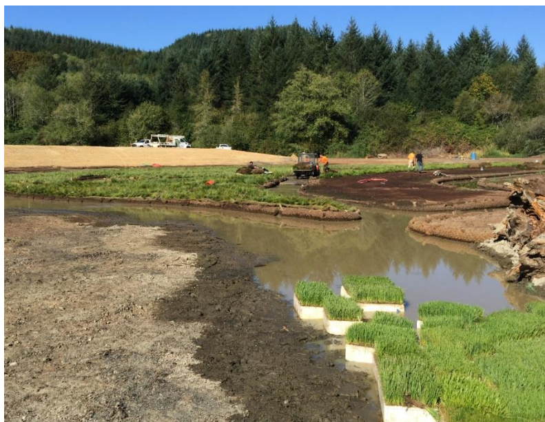
Figure 3-9 Installation of wetland sod
