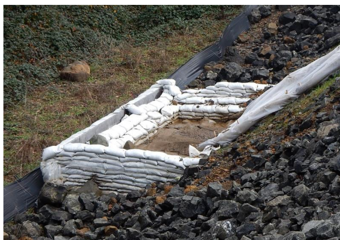
Figure 2-13 Sediment Trap & Energy Dissipater W/ Level Spreader
