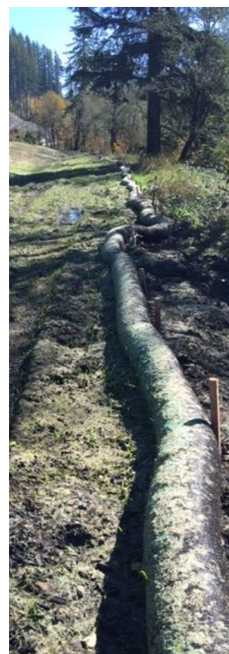
Figure 3-23 Compost Sock – Sediment Barrier Type 8
