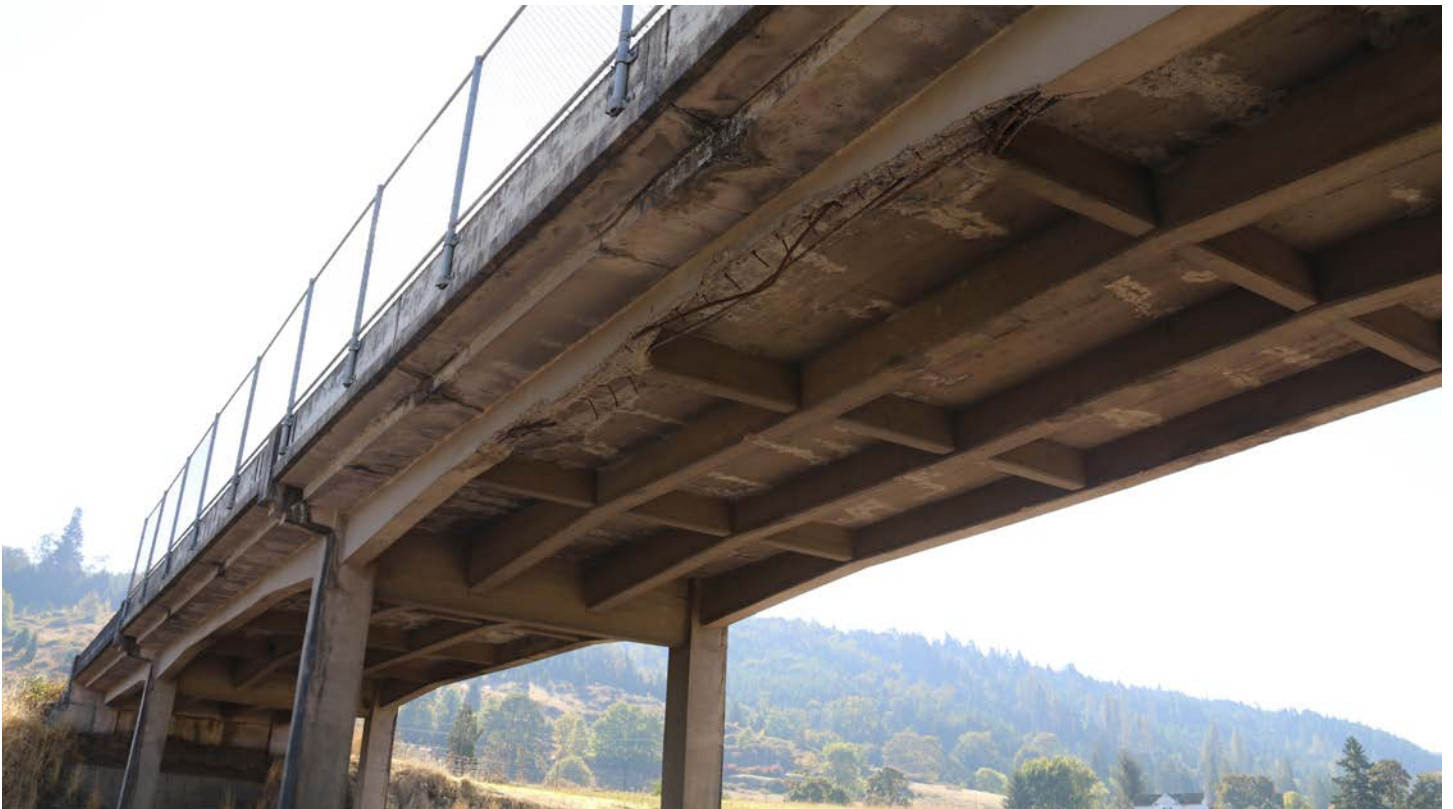
Photo 2: I-5 MP149.39 Equipment Overpass Bridge (Bridge #07643), showing underside of bridge and damage from large vehicles, looking SE (taken 10/4/17 by Kenny Gunn)
