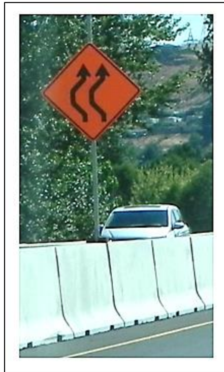
Figure A-4: Concrete Barrier Sign Support
