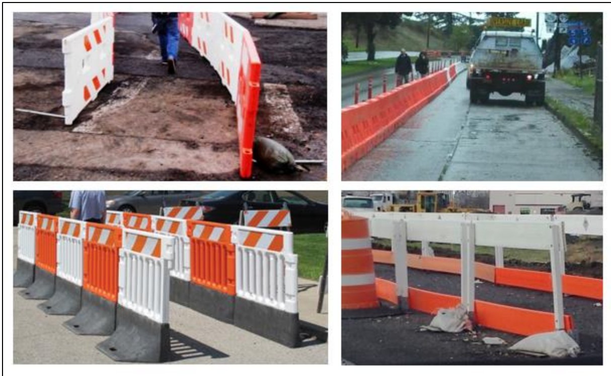
Figure A-1: Pedestrian Channelizing Devices
