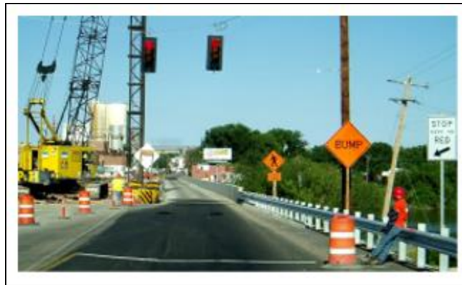
Figure A-1: Temporary Traffic Signal (Span Wire)
