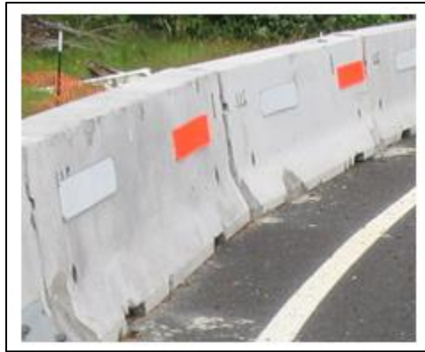
Figure A-1: Reflective Barrier Panels
