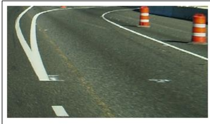
Figure A-1: Temporary Striping for Exit Ramp
