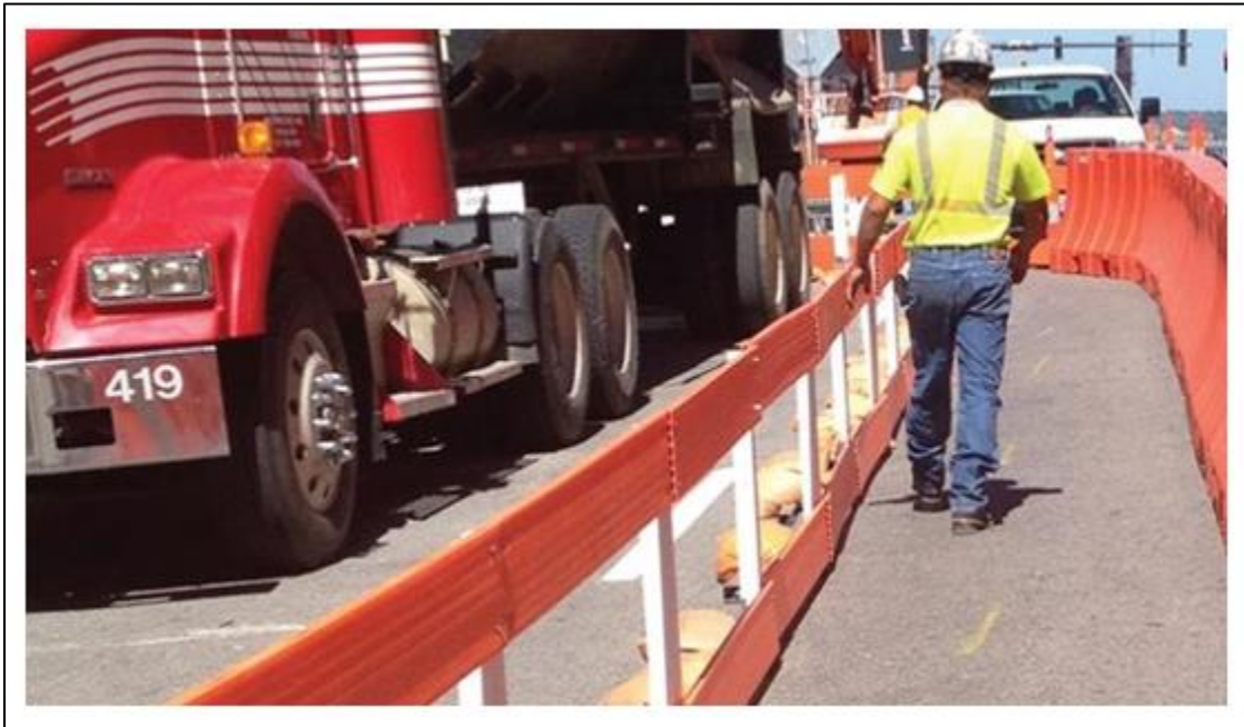
Figure A-4: PCD between Pedestrians and Work Area
