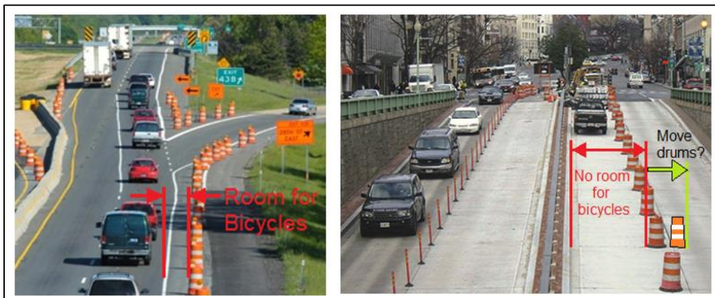
Figure A-4: Shoulder Width Accommodation for Bicycles
