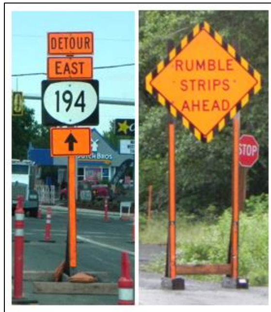
Figure A-2: Temporary Sign Supports
