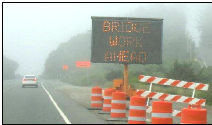
Figure 14 - Rain, fog, smoke, or dust can reduce PCMS legibility.
