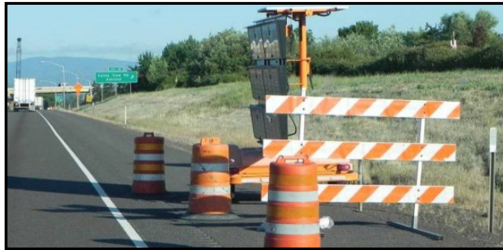
Figure 5 - PCMS lowered and turned away from traffic.
