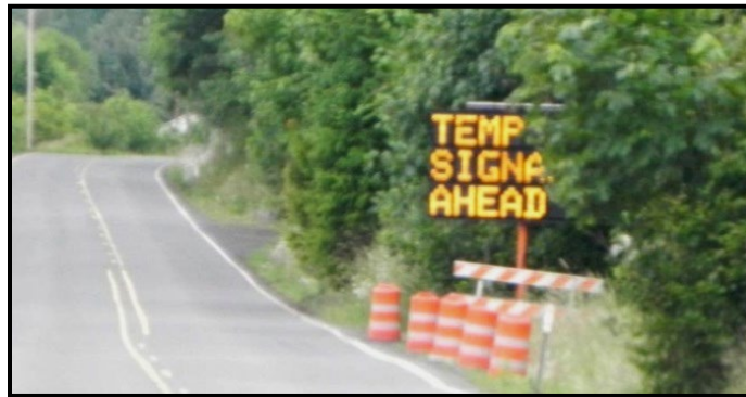
Figure 11 - Field verify PCMS visibility after installation.
