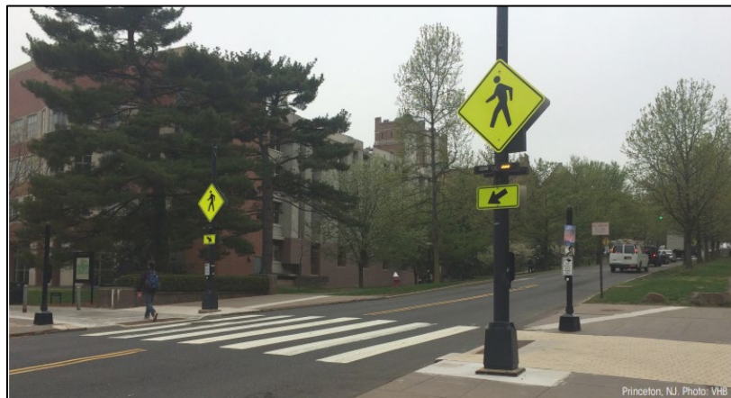
Figure 59. Pedestrian Signal - Rectangular Rapid-Flashing Beacon (RRFB)
