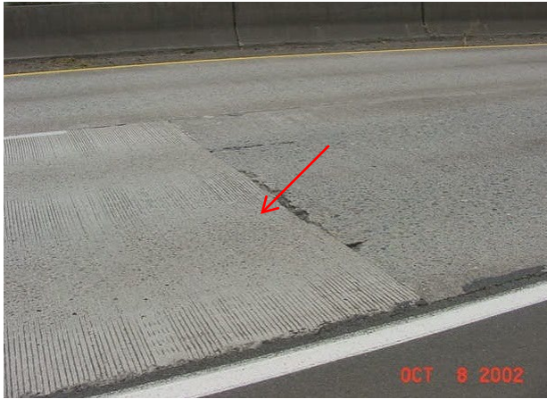
Low – patch is in good condition
