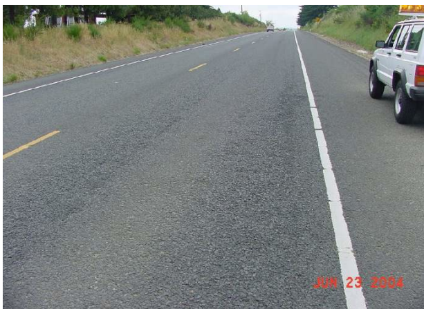
Moderate (both wheel paths, open graded surface)
