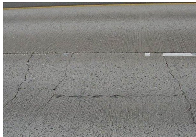
Two low punchouts near centerline
