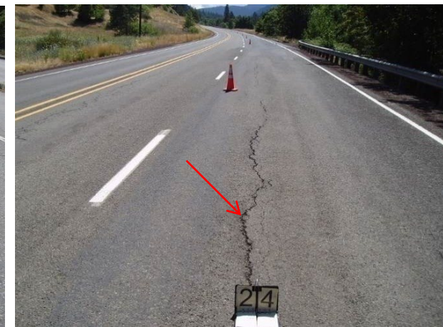
Center – high severity
