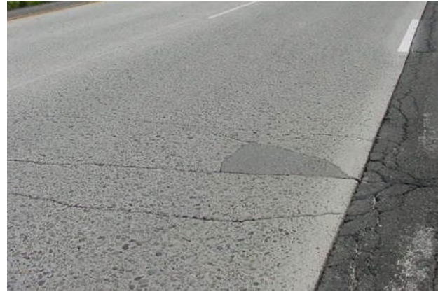
Moderate – irregular concrete patch completely repairing a punchout; record as patch not punchout
