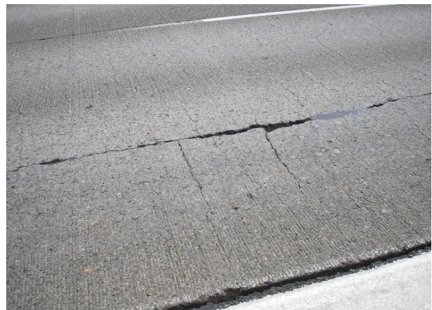
High – right wheel path (based on width)
