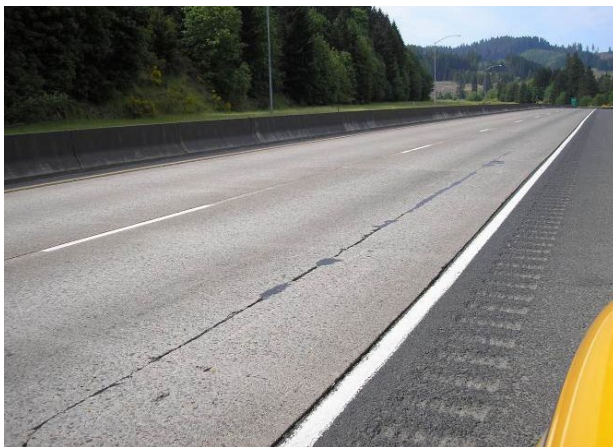
High – right wheel path (based on width and spalling)
