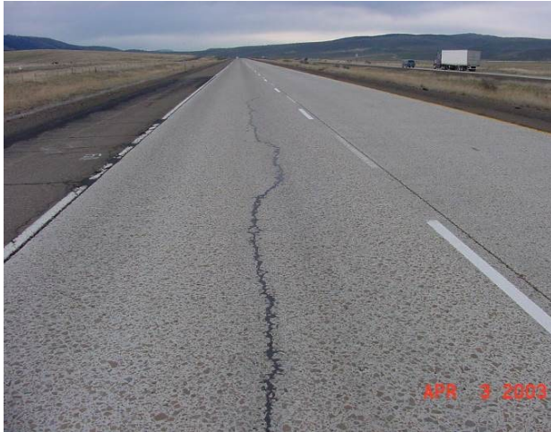
Low – center (based on sealant)
