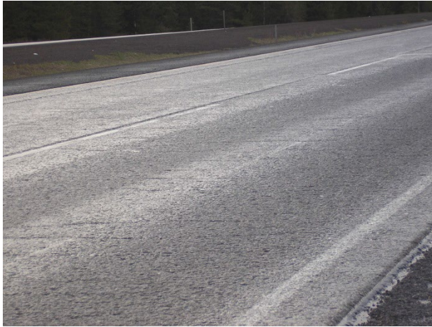
Rough surface may have barely visible longitudinal cracks that should not be rated.
