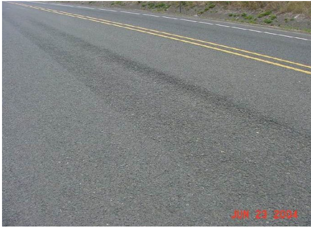
Moderate (both wheel paths, open graded surface)
