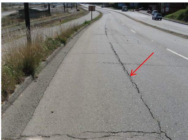
Center – high severity
