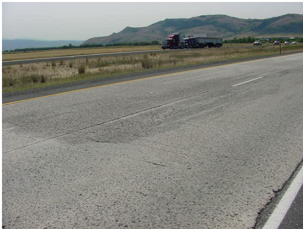
Hairline cracking and scaling should not be rated.
