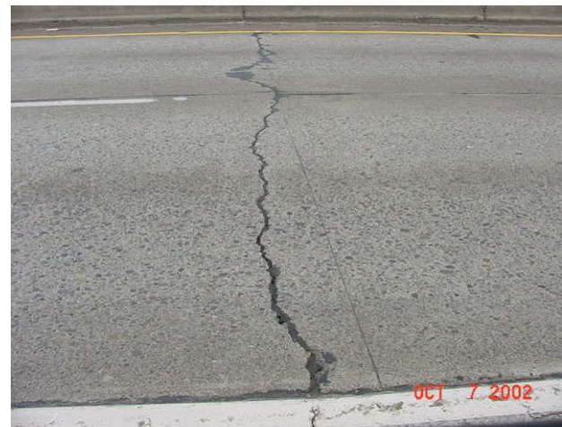
High – transverse crack width is over 1/4"
