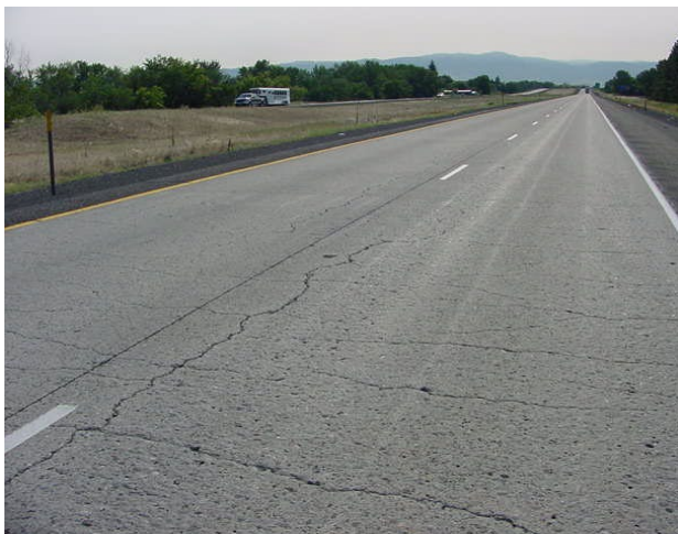
Moderate – left edge (based on width)
