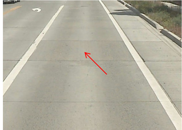
Low – patch has no distress
