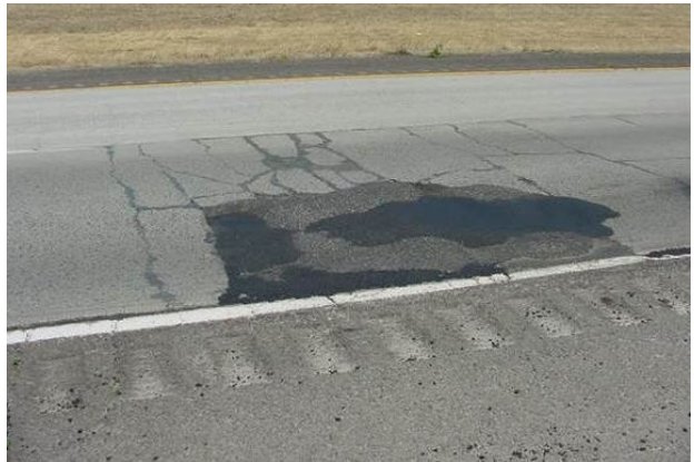
Multiple high severity punchouts covered with high severity patch, this is localized within a single area
