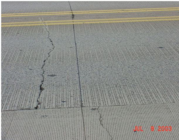
High – transverse crack width is over 1/4"
