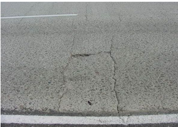
Low – spalling on T-crack and L-crack (if faulted over 0.25”, rate as moderate)
