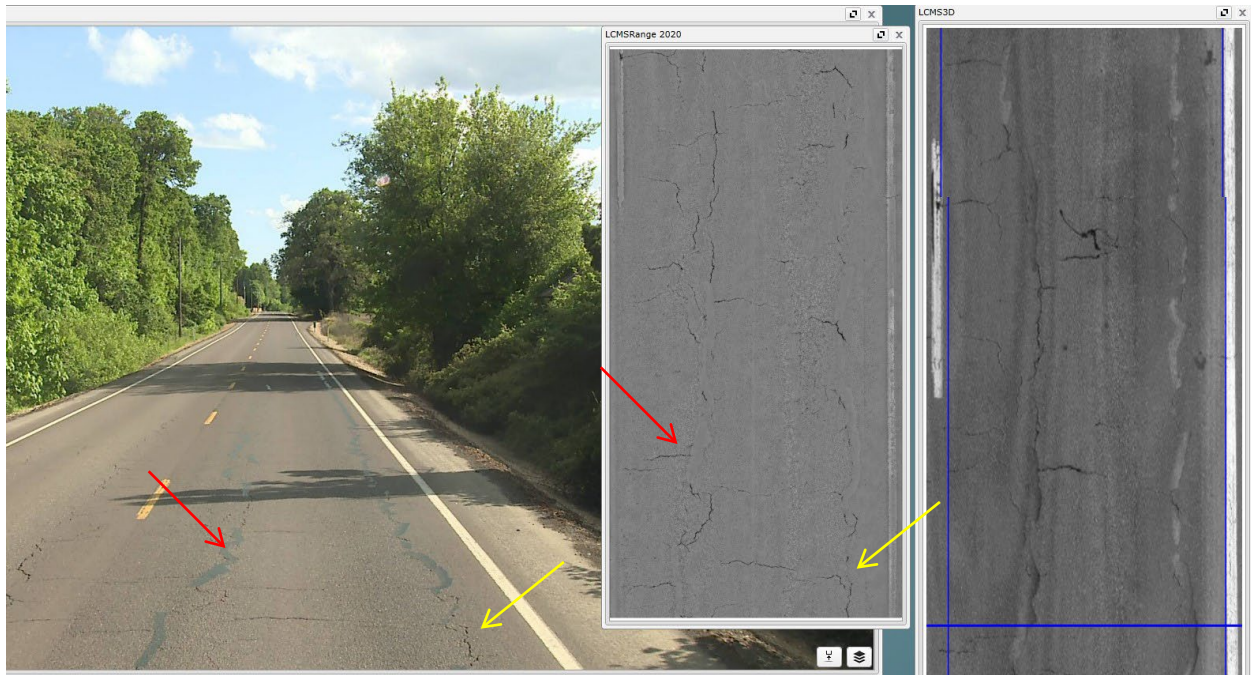
Sealed but open (red arrows) and unsealed (yellow arrows) longitudinal wheel path cracks.
