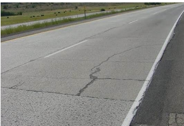
High – patch has spalled transverse and moderate/high severity longitudinal cracks
