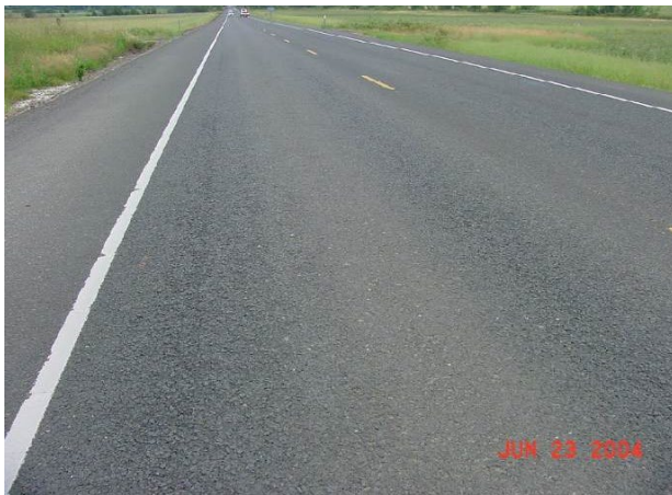
Low in wheel paths (open graded surface)
