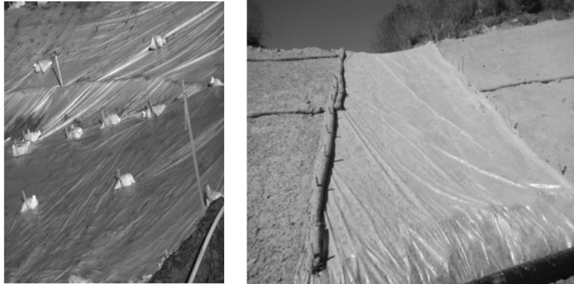
Plastic sheeting 280.44(a) & Standard Detail 6001
