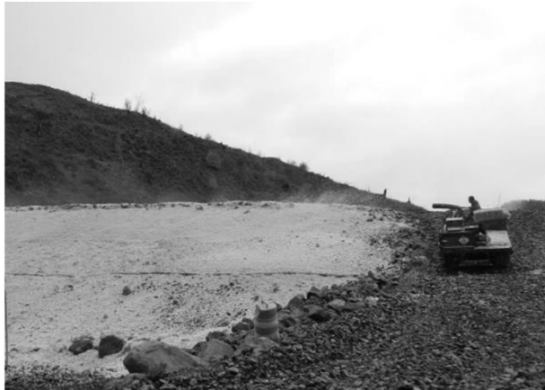
Straw mulch is good temporary cover
