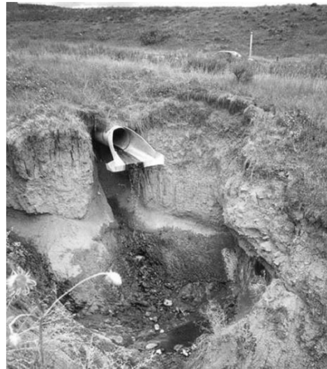
Outfall protection addresses risk
