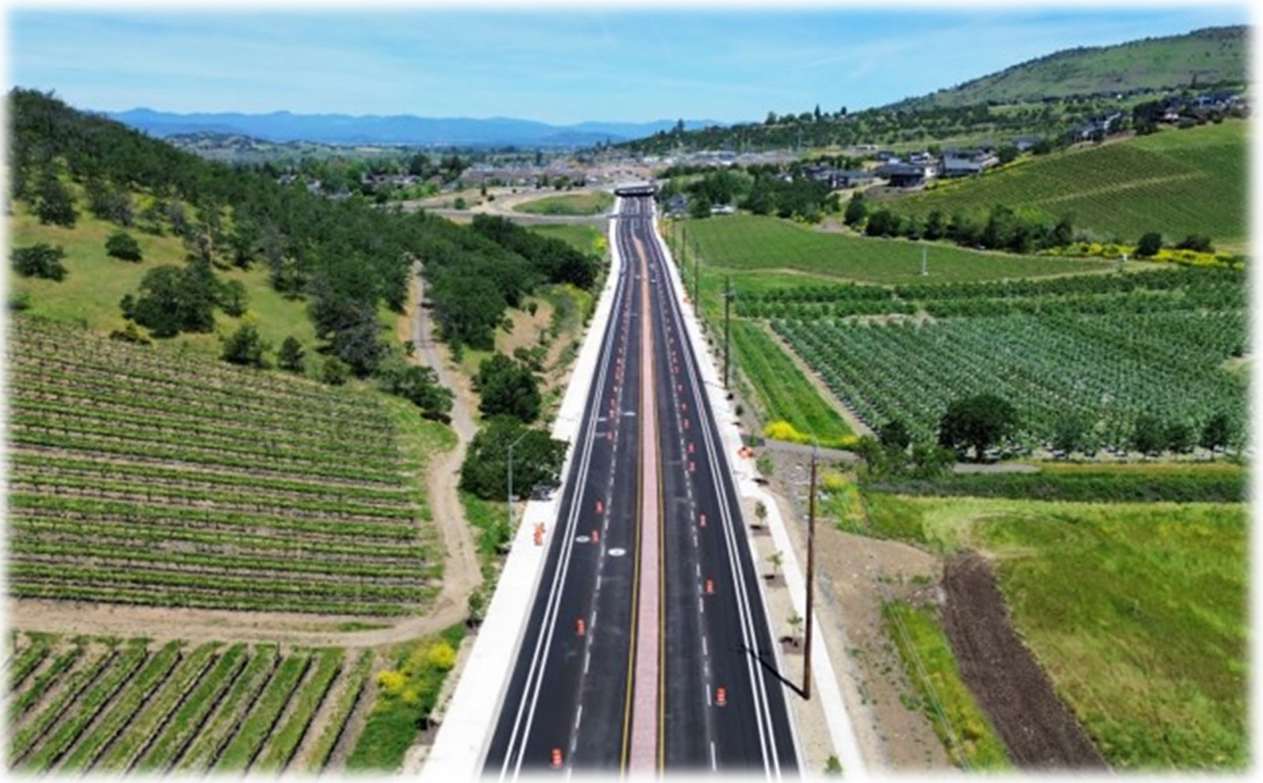
City of Medford, Foothill Road Project
