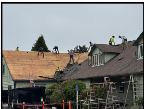
New Roof at Headquarters
