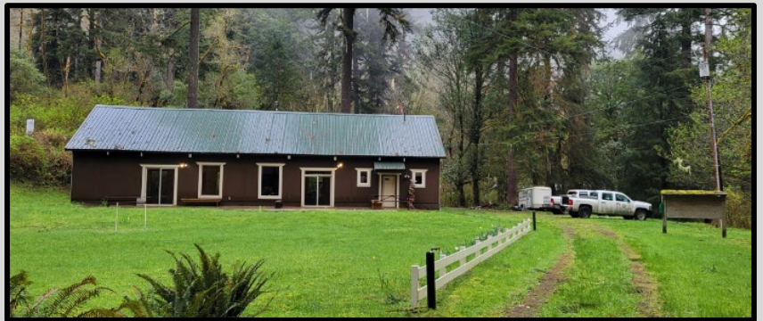
Lodge After Boy Scouts 2015 Renovation
