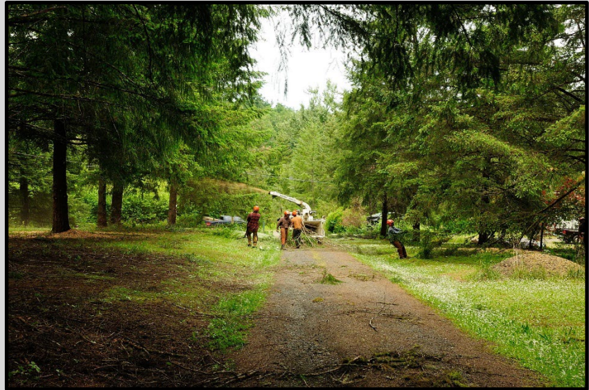
Crew Brushing Landowner's Driveway
