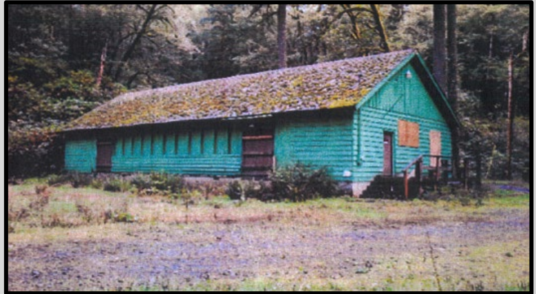
Lodge Before 2015 Boy Scouts Renovation
