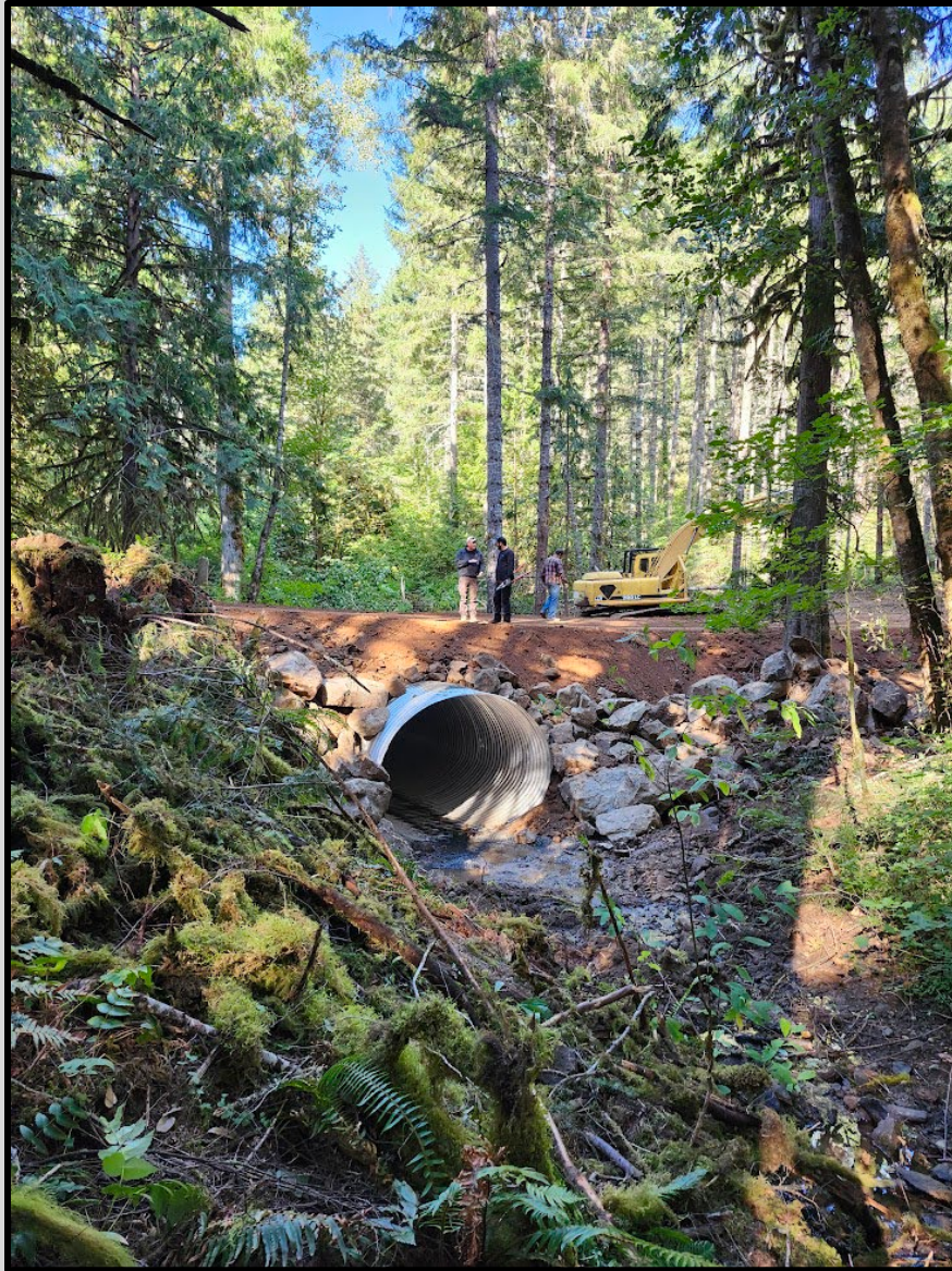
Pipe Installation on M3 Property
