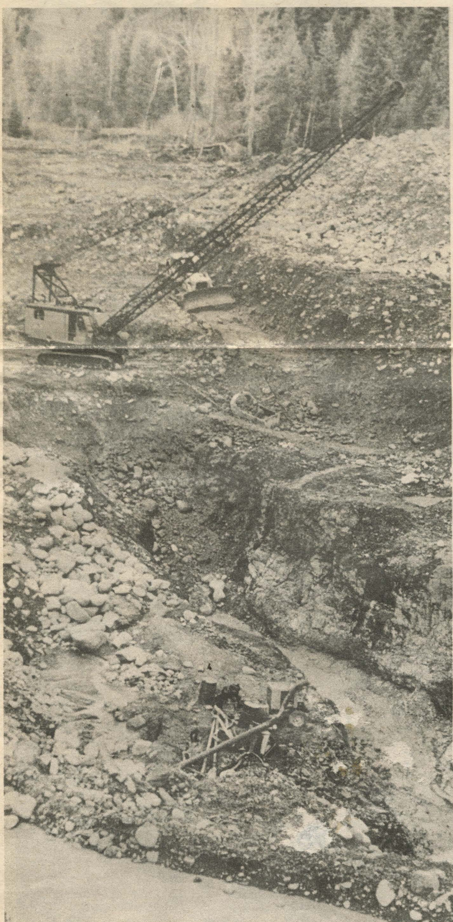
ALTHOUGH the Cornucopia Minerals Inc., mining operation requires digging deep into the earth adjacent to Pine Creek, state regulations will require the miners to fill in the hole and cover the area with topsoil so it will again grow trees and grass. A previous mining operation left boulders and gravel atop the ground which prevented anything from growing.
