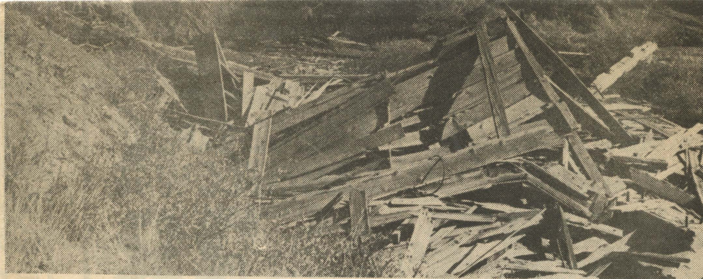
The depression in the center of the picture is the main shaft of the Bonanza, extending down into the mountain 1250 feet, "the deepest shaft in Eastern Oregon," the 1903
