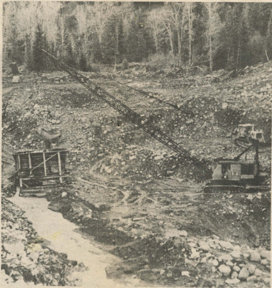
CRUDE GRAVEL is scooped up by the drag line up to three cubic yards at a time. The miners are working in a narrow valley below the old Cornucopia mine about six miles north of Halfway. This area had been previously worked, but gold for jewelry manufacturing is expected to make the operation profitable.
